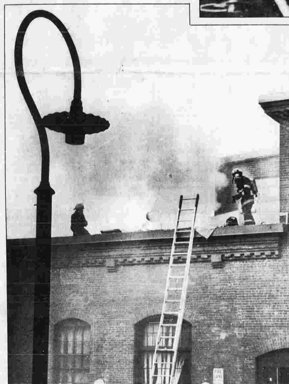
BATTLING THE BLAZE — Town of Manchester firefighters are working around a hole put in the roof, while others look on, at the site of a fire in the Clocktower Mill Apartments this morning. The fire caused smoke and water damage in at least two apartments of the 185-unit complex.
